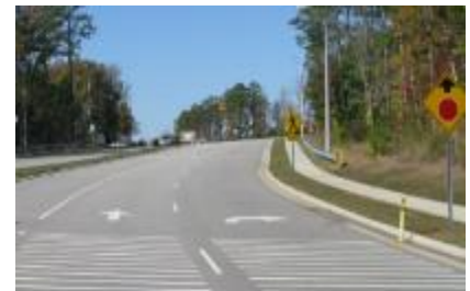
Figure 20 Example of transverse rumble strips applied along a multilane. Source: VHB
