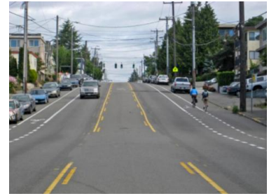
Figure 19 Example of lane narrowing, creating space to install bike lanes and a buffer for pedestrians. Source: PEDSAFE
