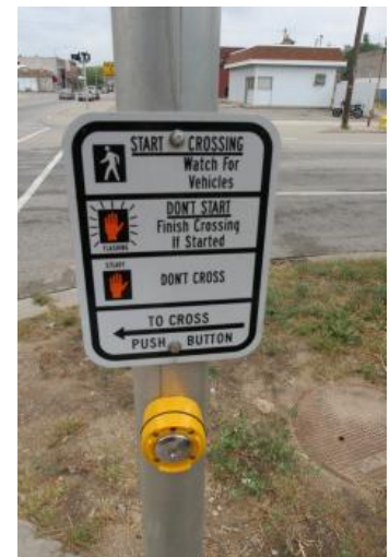
Figure 24 Example of a pedestrian push button, allowing pedestrians to activate the crossing signal. Source: PEDSAFE & FHWA
