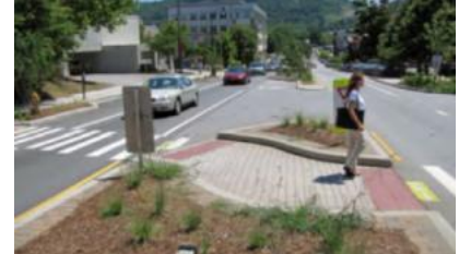
Figure 14 Example of a right-turn slip lane with a raised landscaped median. Source: Living Streets, PEDSAFE
