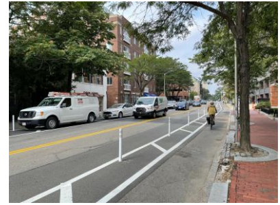
Figure 15 Separated bike lane on an urban two-lane roadway. Source: City of Cambridge.
