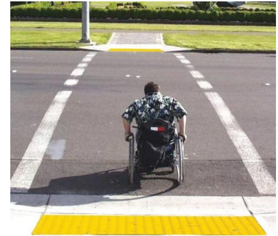
Figure 9 Example of curb ramp accessibility for restricted pedestrians. Source: FHWA
