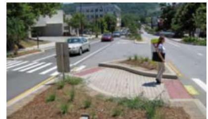
Figure 14 Example of a right-turn slip lane with a raised landscaped median. Source: Living Streets, PEDSAFE
