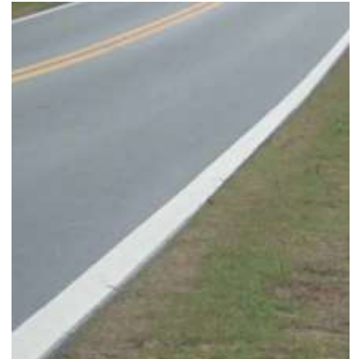
Figure 13 Application of 6-inch-wide edge line. Source: Texas Transportation Institute
