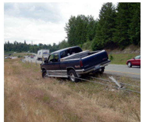
Figure 18 Median cable prevents a potential head-on crash. Source: WADOT
