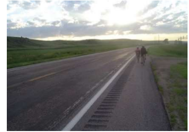
Figure 1 Example of paved shoulders with rumble strip separating motorists from bicyclists. Source: BIKESAFE
