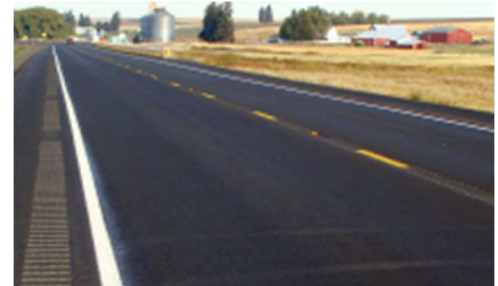
Figure 16 Shoulder rumble strip and center line rumble strip. Source: FHWA
