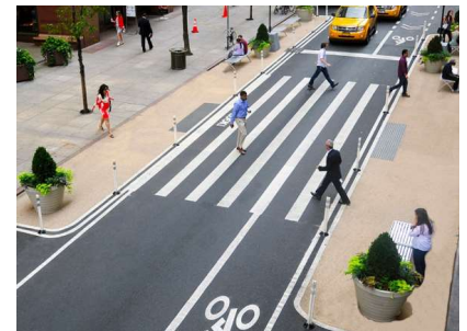
Figure 12 Example of mid-block narrowing in Manhattan. Source: NYCDOT
