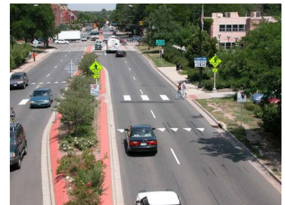
Figure 14 Advanced yield markings at a midblock crosswalk with a refuge island. Source: pedbikeimages.org - Toole Design Group
