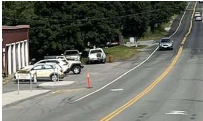
Main Street / US-302 at the Intersection of Maia Papaya and Post Office East entrance.
