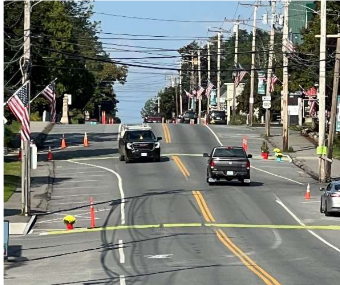
Town Hall Crosswalk
