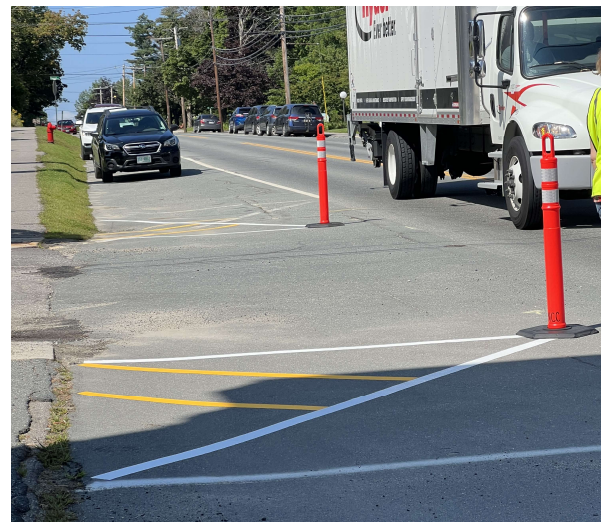
Main Street / US-302 at the Intersection of Jefferson Street
