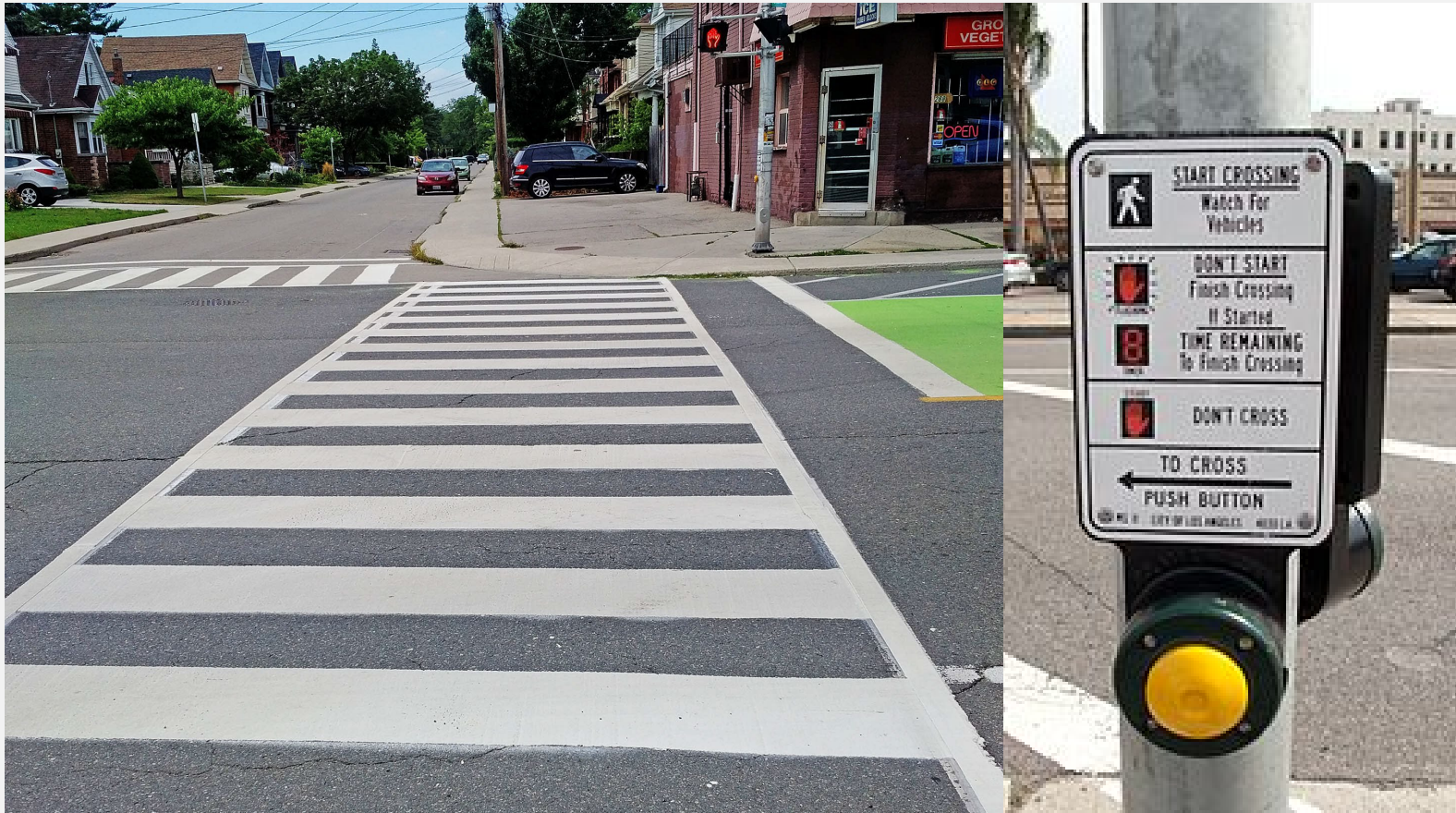
Controlled pedestrian crossing
